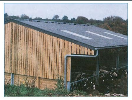
Figure 24: The upper wall cladding should cast a shadow line over the lower plinth
