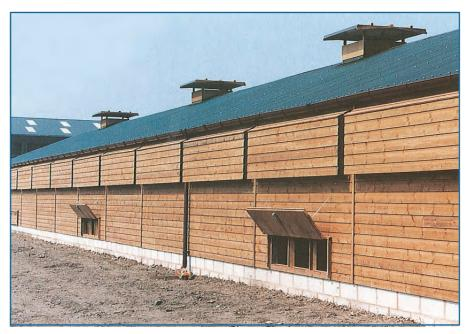
Fig 19: Example of horizontal timber, 'lapped' feather-board cladding
