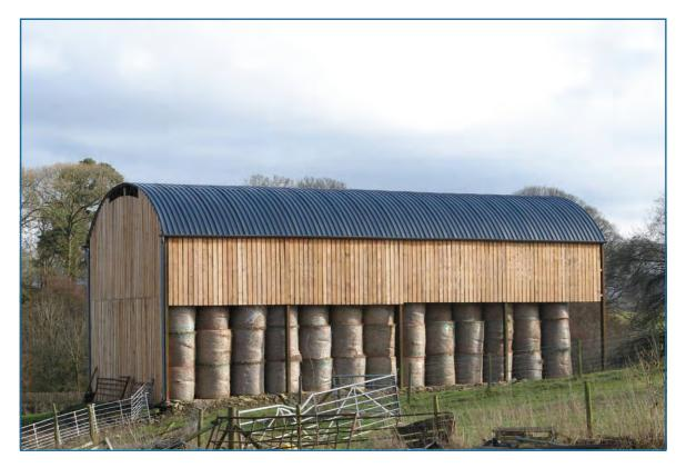
Figure 4: New Dutch barn constructed from timber
