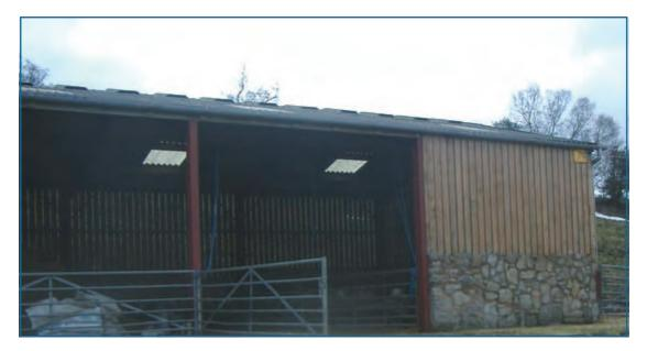
Fig 23: Conspicuous plinth walls should be clad with timber or stone
