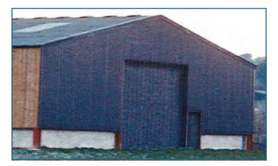
Fig 26: Example showing recessed machine and pedestrian doors in large building
