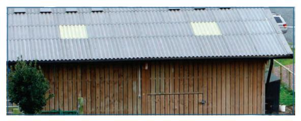
Figure 22: Overlapping Eaves should project to the maximum
