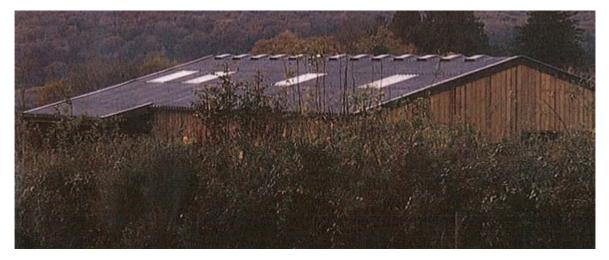
Fig 21: Fibre cement roofs are the least reflective roof material
