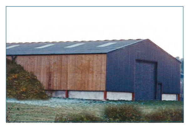
Figure 25: Example of a building showing contrasting colours used on elevations to break up building profile. A dark coloured solid cladding on one face of the building and Yorkshire board on an adjacent face reduces the apparent size of the building.
